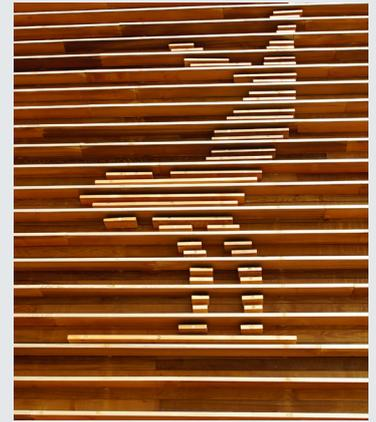
**Facts:** WRC panels impregnated with Woodsafe Exterior WFX for natural aging with no other surface treatment required.
