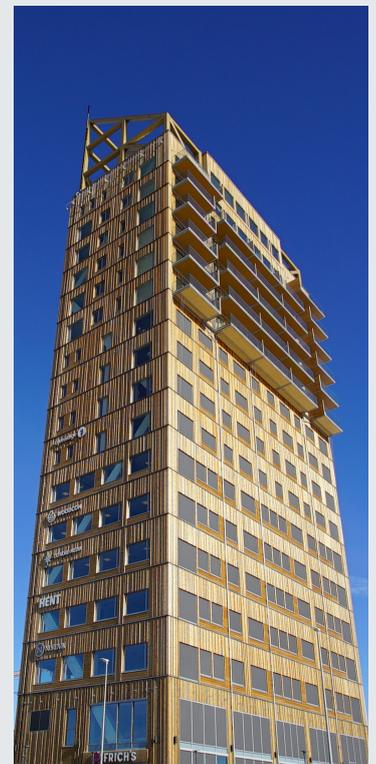
**Facts:** Exterior cladding of Thermowood-D impregnated with Woodsafe Exterior WFX.
