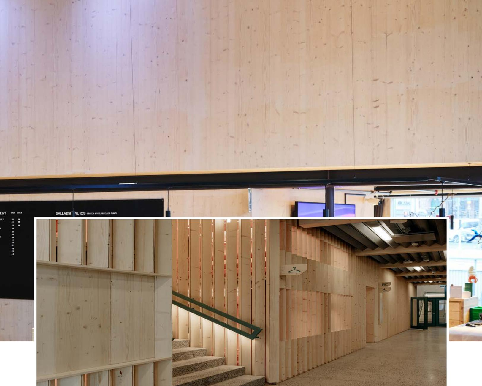
**CL BOARD** is a building component consisting of at least 3-5-7 layers of glued boards or planks made of softwood, where every second layer is at 90 degrees to the adjacent layer.
