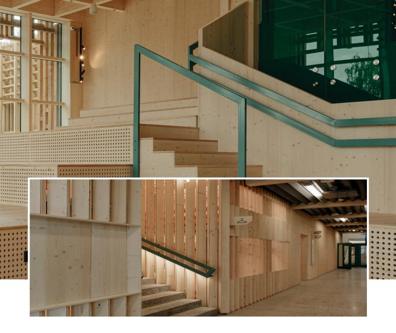
**CL BOARD** is a building component consisting of at least 3-5-7 layers of glued boards or planks made of softwood, where every second layer is at 90 degrees to the adjacent layer.
