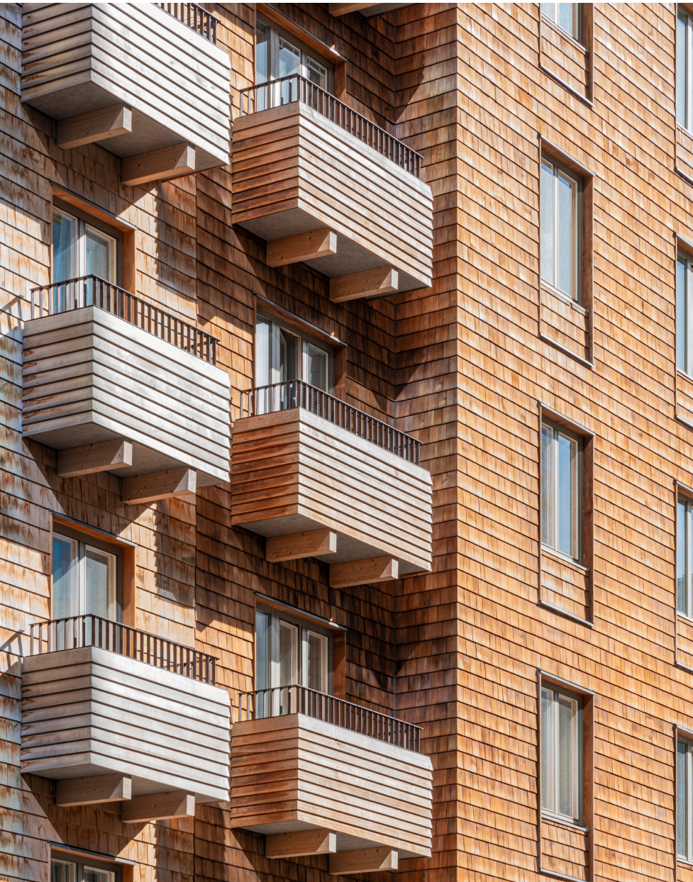
Picture shows Cederhousen with cedar shingle, fire retardant treated with WOODSAFE Exterior WFX. Credit to: Michael Perlmutter
