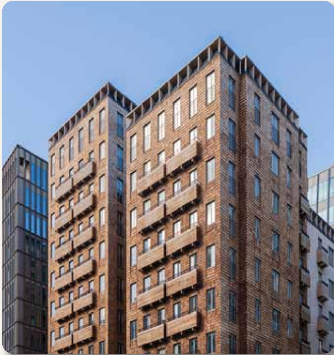
Western Red Cedar shingles and Yellow Cedar (SP Fire 105 + EN 16755 EXT)
